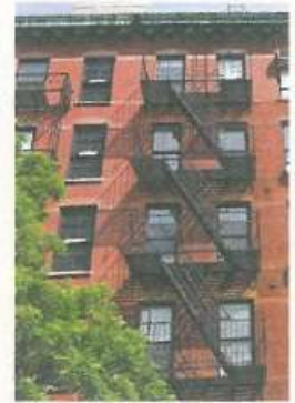
6 a fire escape
